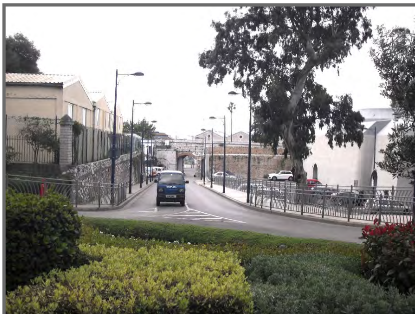
Figure 2.7 – Ragged Staff Pedestrian Crossing (Before)
