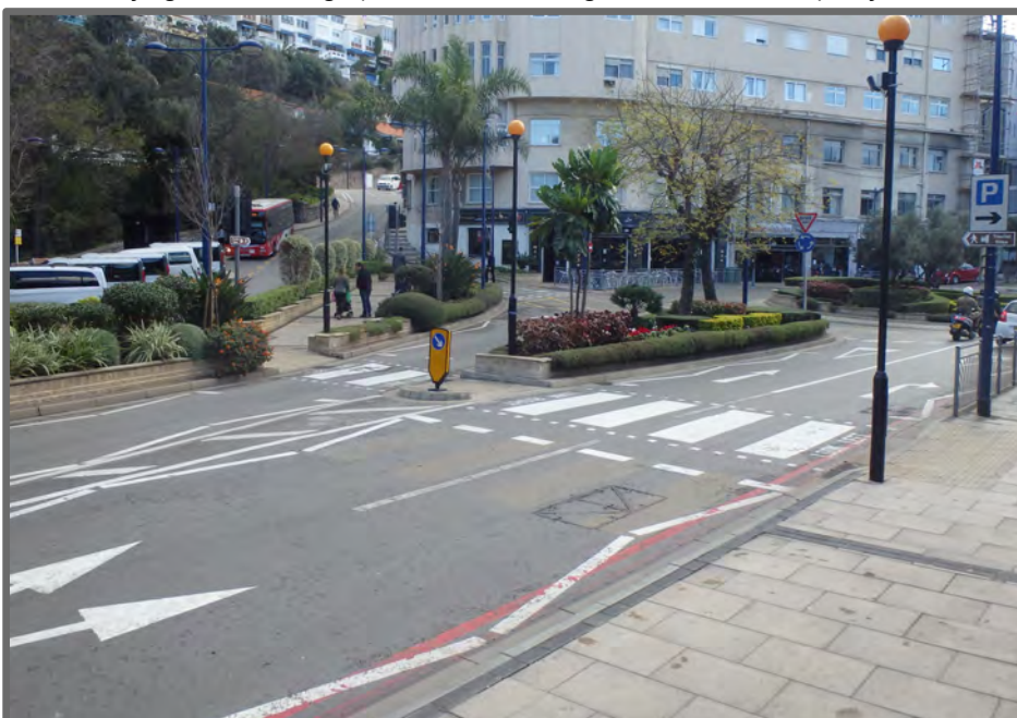
Figure 2.2 –Trafalgar Interchange (Pedestrian Crossing with Centre Island) – After
