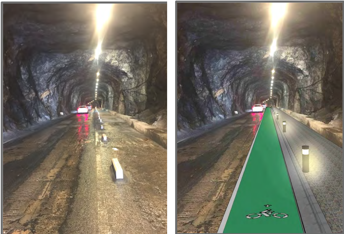
Figure 2.11 – Keightley Way Tunnel (Pedestrian Route Enhancement) – Before and after
