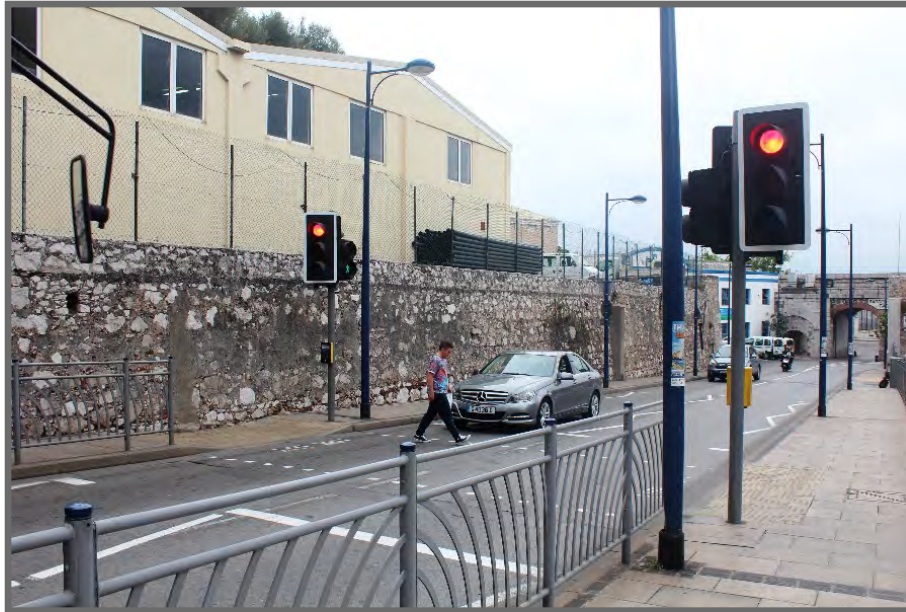
Figure 2.8 – Ragged Staff Pedestrian Crossing (After)
