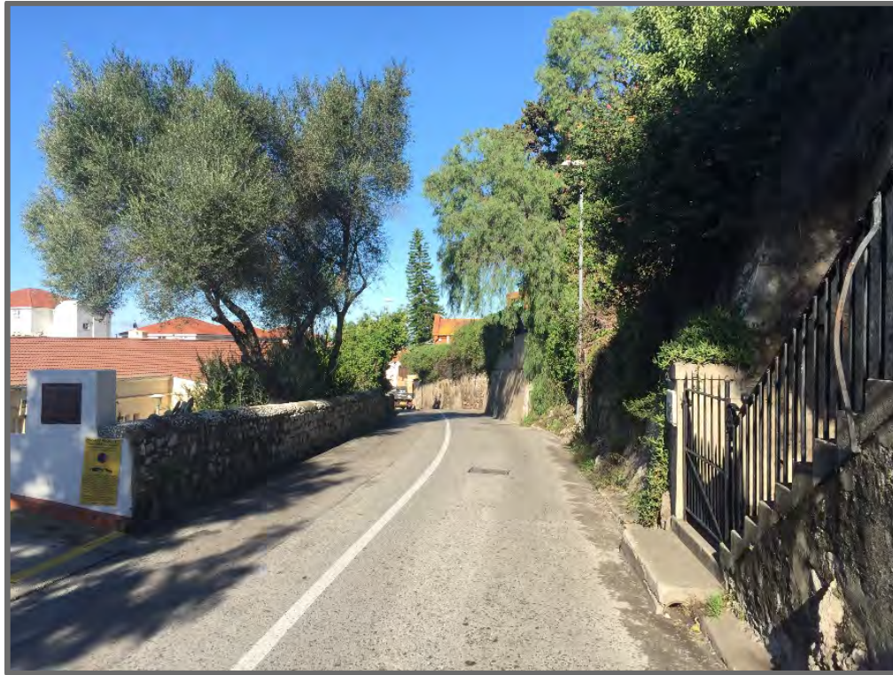
Figure 4.6 – Europa Road (Section considered for Widening)
